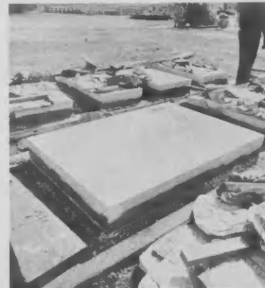
This is not a graveyard, but completed panels drying in the sun.
